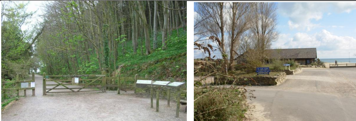
Boundary treatments should relate to the local environment Above left: Simple timber post and rail fencing at National Trust Car Park at Golden Cap (photo Halcrow) Above right: Local stone used in the National Trust Car Park at Studland (photo Halcrow)
