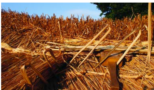
Thatching the ridge of a roof.
